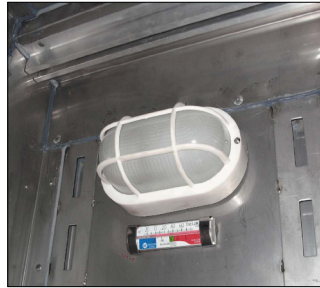
Internal lighting dual voltage source 115/230 VAC
